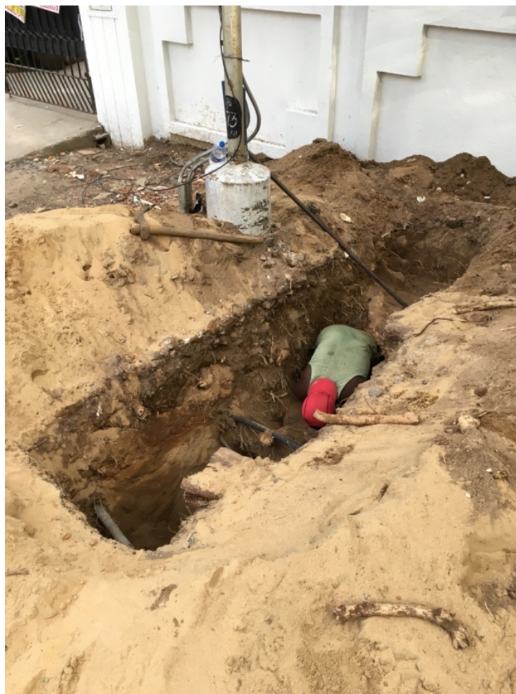
Figure 24. Digging in Besant Nagar, July 2018. Photograph by the author.
