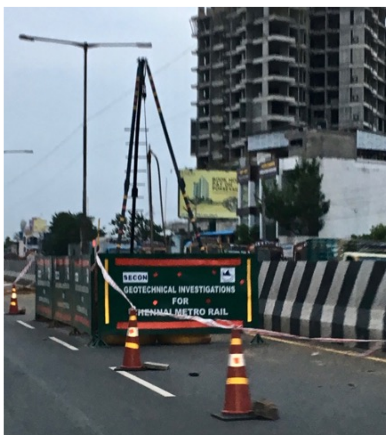
Figure 35. Geotechnical Investigations at Kolathur, Chennai, July 2018. Photograph by the author.
