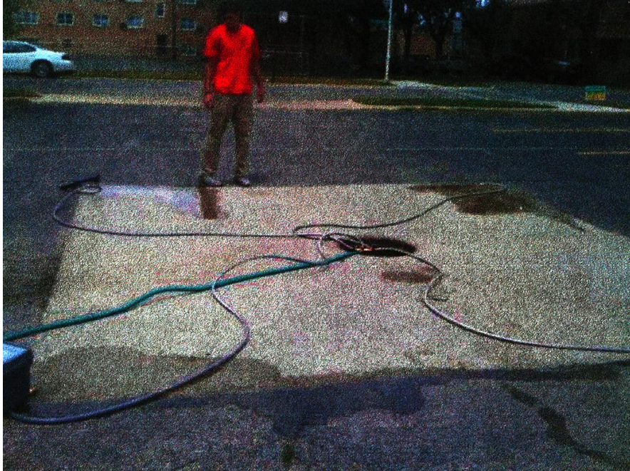
Figure 7: Configuration of Hoses on West Permeable Pavement Section
