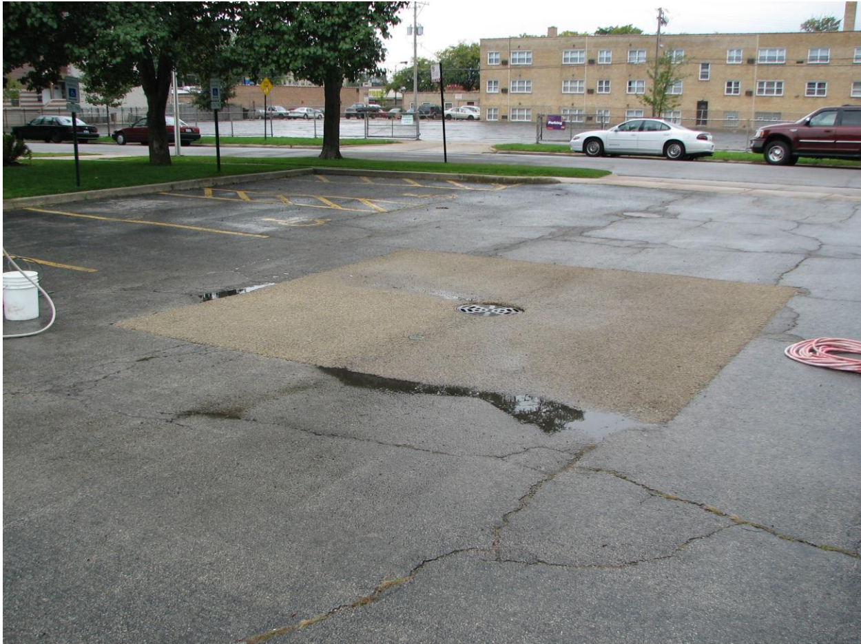
Figure 2: A Permeable Pavement Patch at St. Margaret Mary Parish
