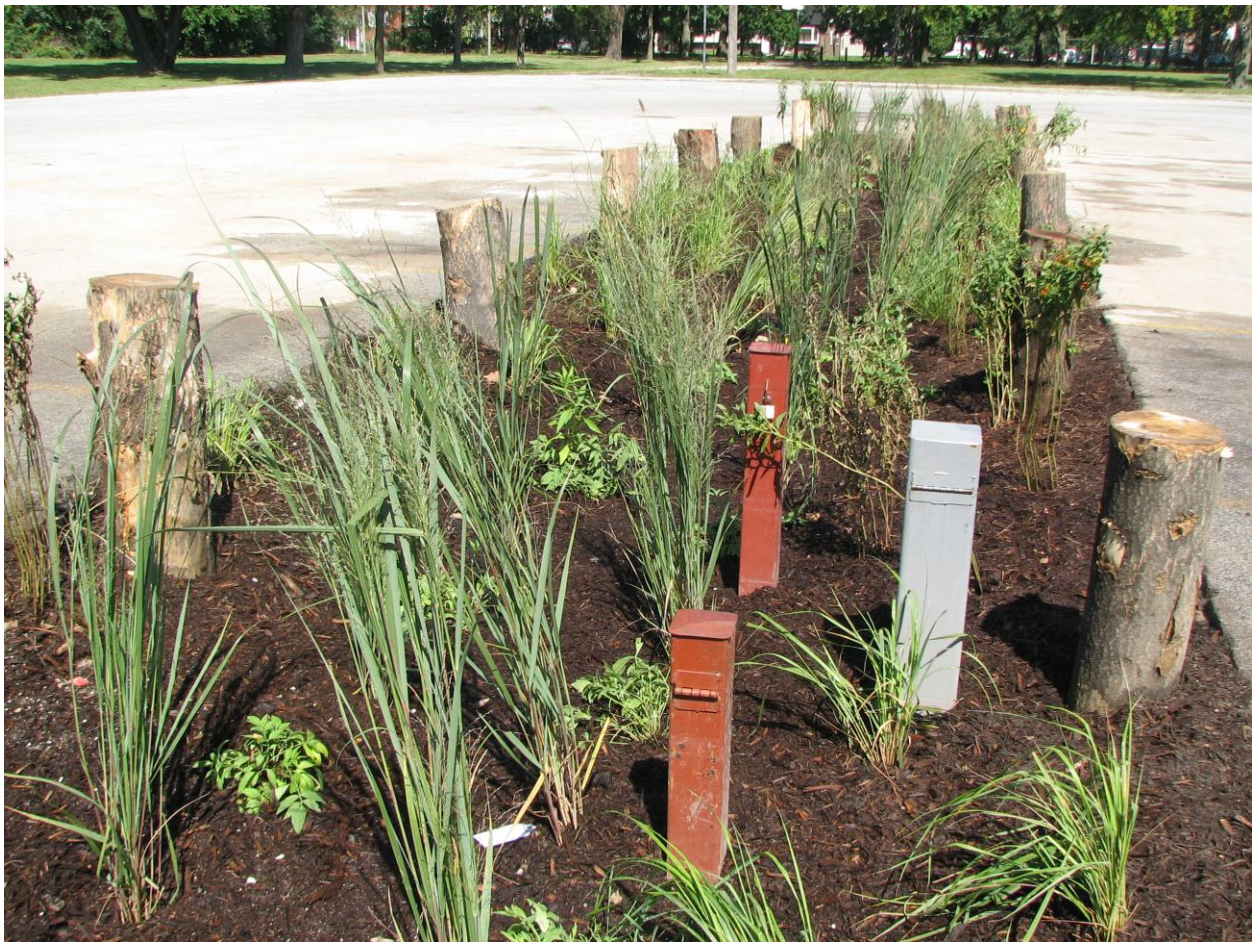
Figure 1: Details of the Bioswale at Our Lady Gate of Heaven Parish, including three monitoring wells
