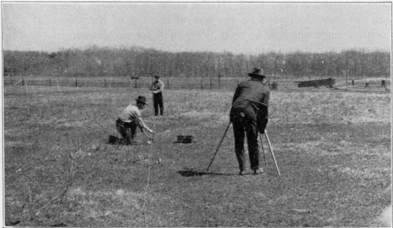
FIG. 12.—USING A DRAINAGE LEVEL TO STAKE OUT THE TERRACE
