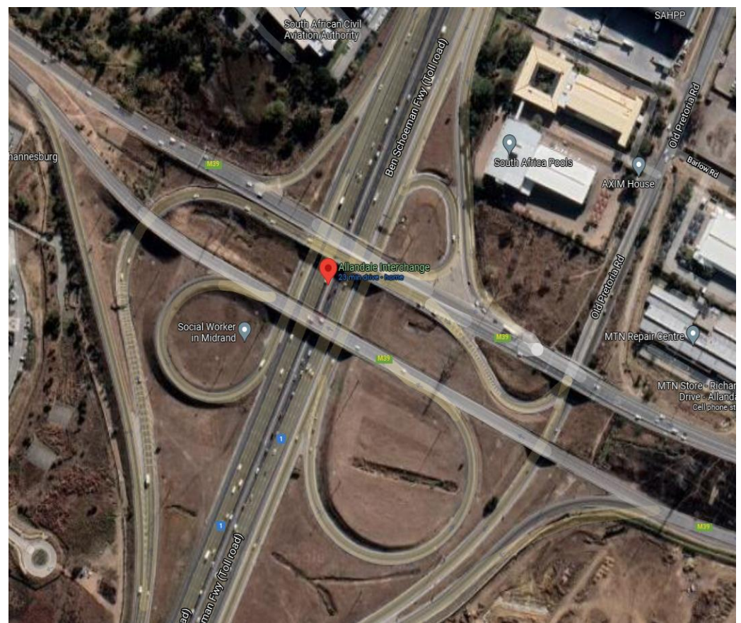
Figure 3. The road intersection (Allandale Interchange).
