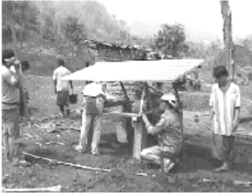
Picture 7. Installation of solar modules
