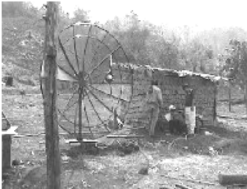
Picture 5. Installation of a C band antenna
