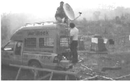
Picture 4. Installation of a Ku band antenna
