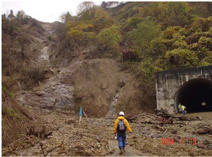
(b) Gravels obstructed the portal entrance in Sinotani tunnel
