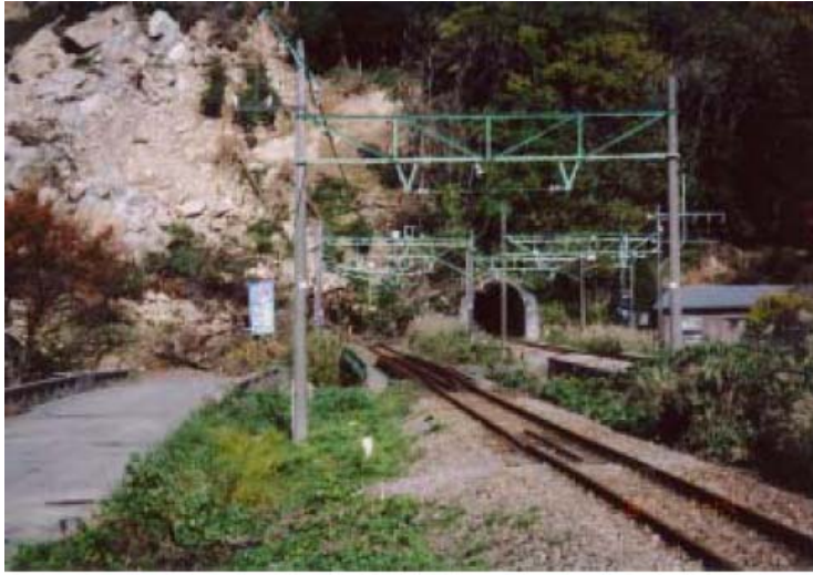
(a) A landslide obstructed the portal entrance in Enoki tunnel
