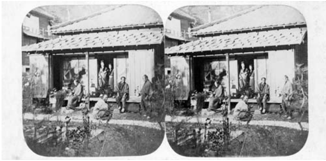
Fig. 8 Pierre Rossier: 'Jeda. [Tokyo] Group of Japanese, and general construction of a Japanese Dwelling.' No.61, 1859, albumen-print stereoview, 83 x 174mm
