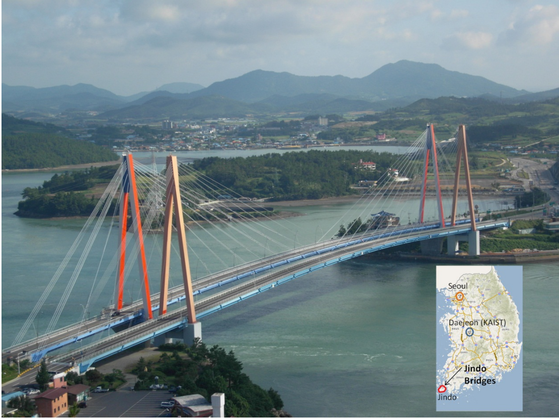
Figure 9.7: Twin Jindo Bridges connecting Jindo Island with the Korean Peninsula.
