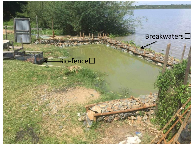
Figure 11 New breakwaters and the previous bio-fence.
