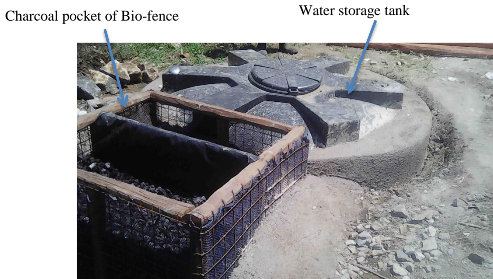
Figure 12. The new Bio-fence under the construction
