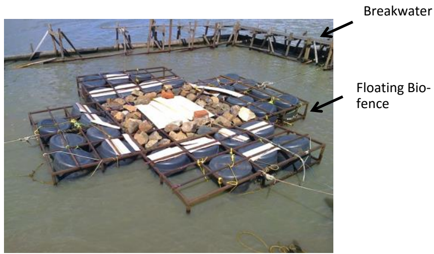
Figure 2. The floating type Bio-fence protected by the breakwater made of timber plates and poles.
