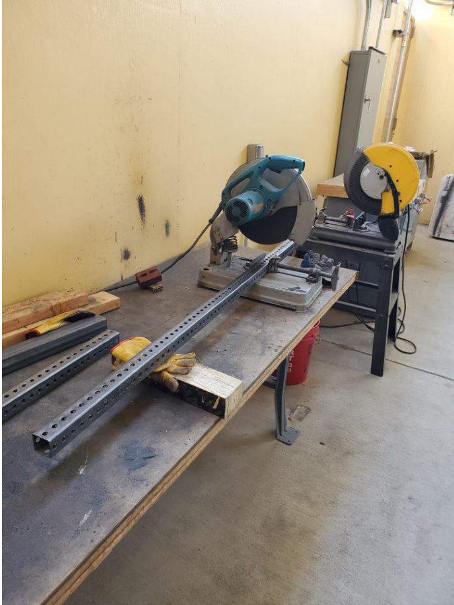
Figure 34. Steel Bolt Together Framing and Fitting Cutting Set-up
