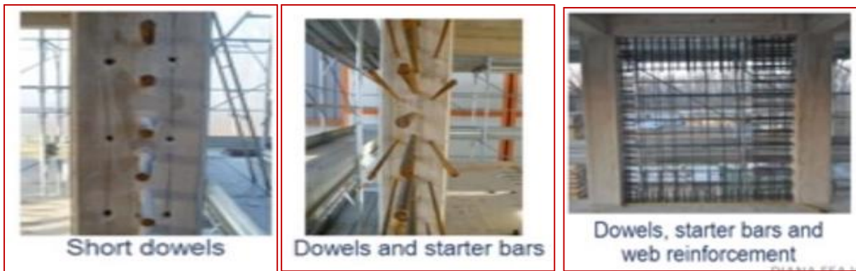
Figure 11. (a) Short dowels, (b) starter and dowels bar, (c) Starter, dowels and web bars
