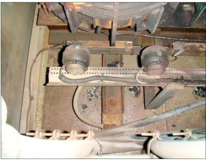
Figure 1. The results of salt laden air being drawn into the transformer enclosure
