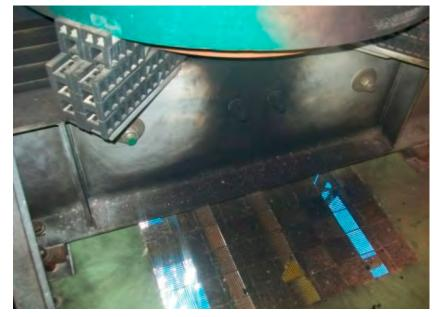
Figure 4. The effect of generator exhaust gases entering the transformer enclosure from the deck below on a drilling rig
