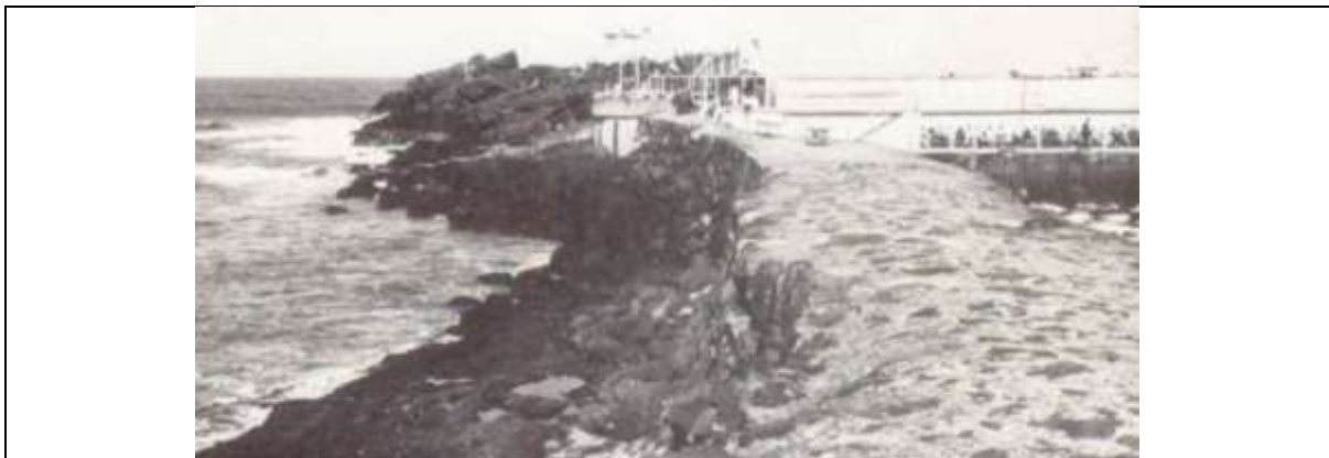
Figure D.6 North Berwick breakwater
