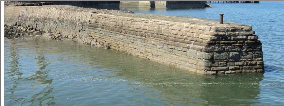
Figure D.4 Cockenzie West Breakwater, May 2013
