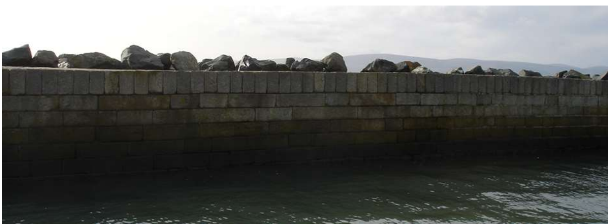
Figure 2.4 Inner face of Dublin Great South Wall
