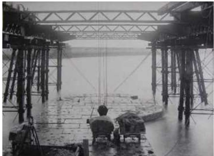
Figure 12.11 Dover - placing concrete blockwork from travelling cranes
