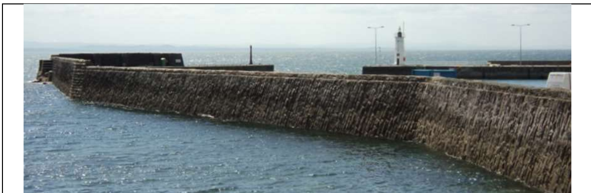
Figure D.1 Anstruther main (East) breakwater, July 2013
