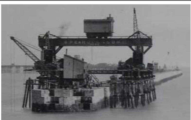
Figure 4.5 Dover - placing blockwork from travelling cranes Courtesy Dover Harbour Board
