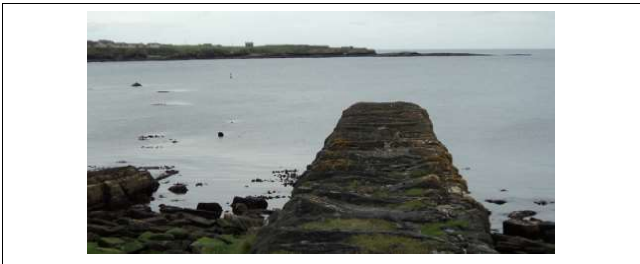
Figure 2.27 Remains of Stevenson's pier, May 2014
