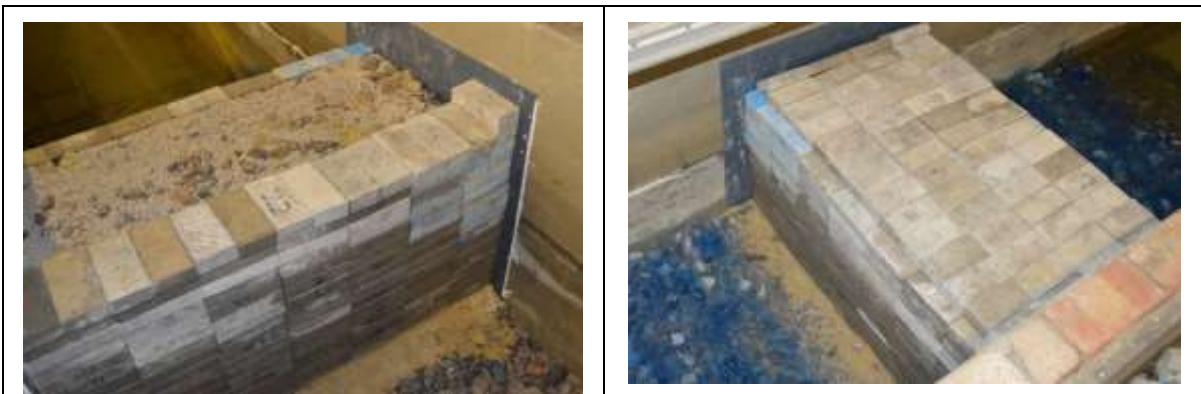
Figure 7.17 Crest protection for Series 3, a) bedding layer for crest; b) crest blocks
