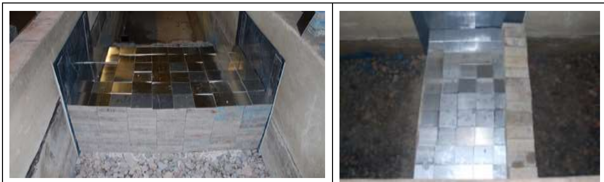
Figure 7.26 Test section for Series 5, showing crest slabs and parapet wall
