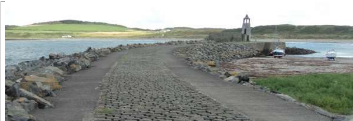
Figure D.1 Repaired mole and lighthouse at Port Logan (W. Allsop, 2017)
