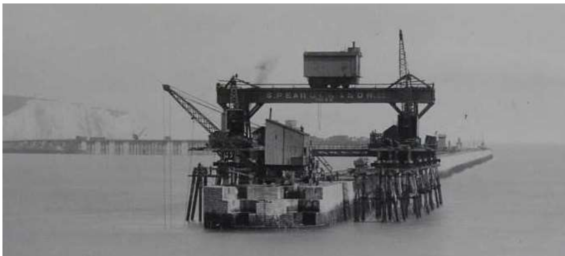
Figure 2.36 Construction of South Breakwater using Goliath crane on staging
