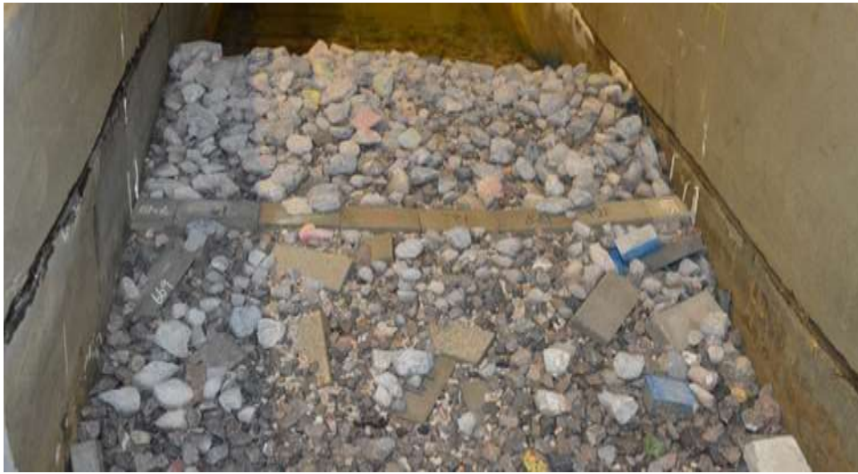
Figure 7.13 Series 2, post collapse, view from seaward
