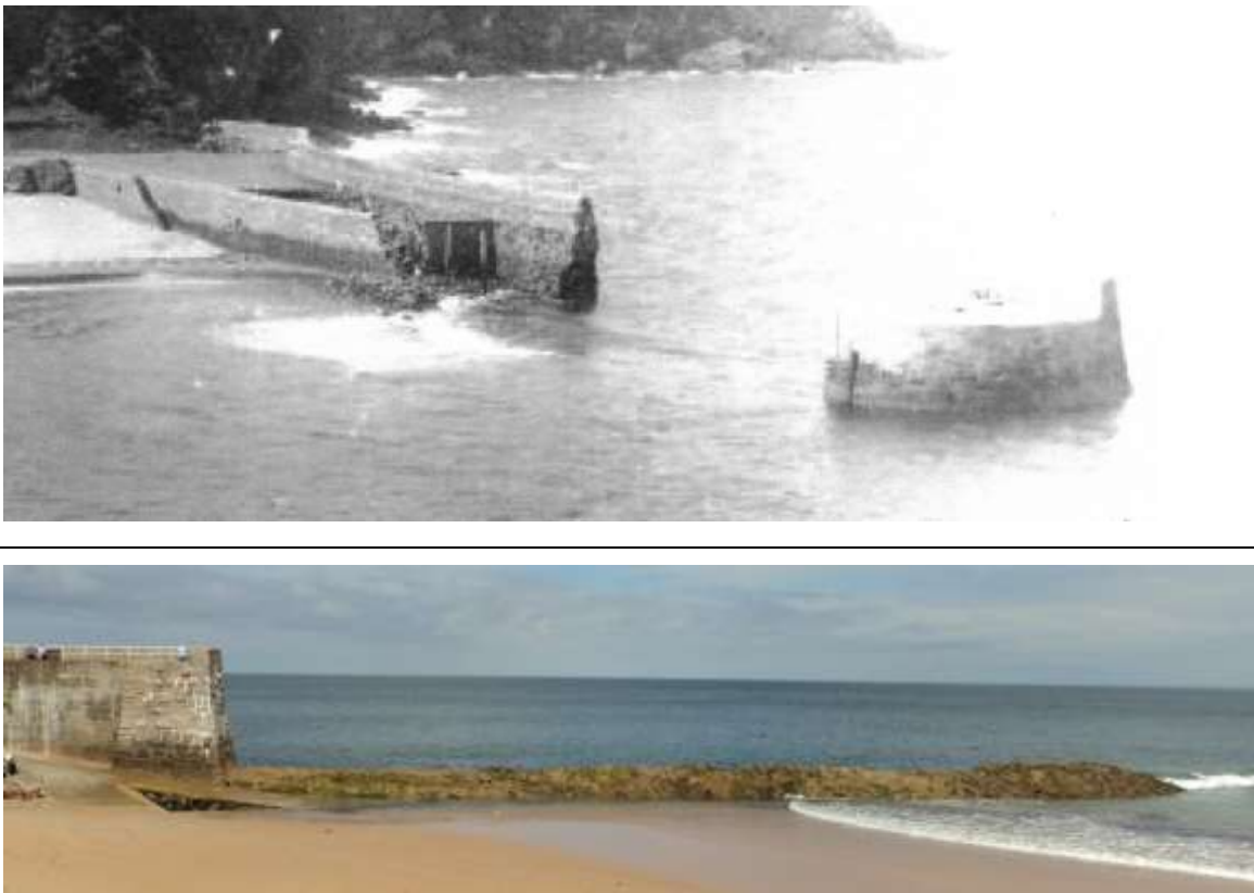
Figure 2.32 Failure at Greve du Lecq, Jersey, 1884
