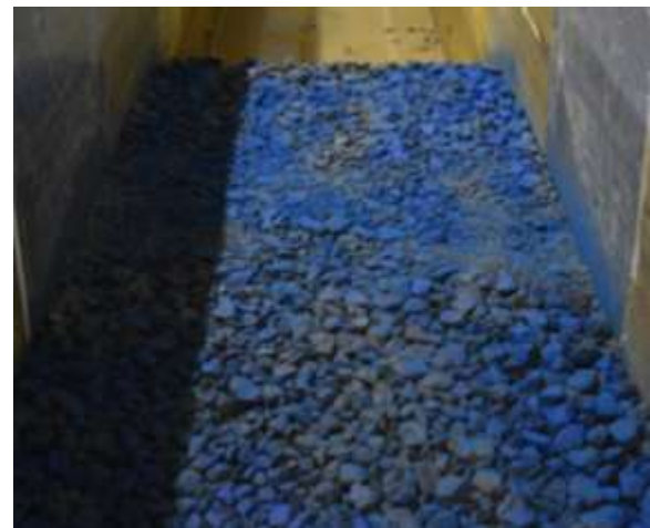
Figure 7.5 Rubble mound platform before wall construction
