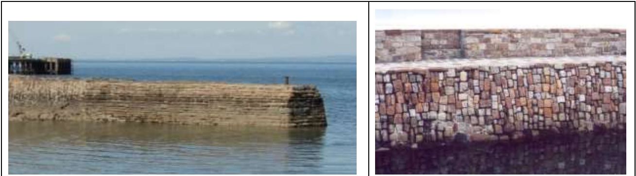
Figure 3.12 Variable blockwork placement at: a) Cockenzie; b) St Andrews
