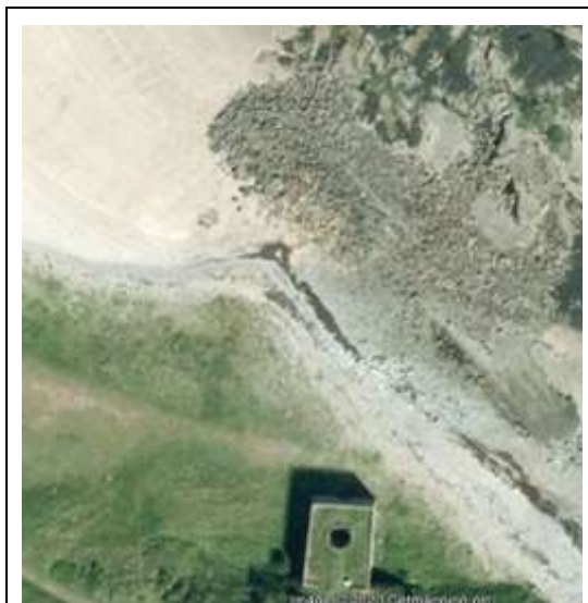
Figure 2.29 Collapsed breakwater and limekiln at Skateraw
