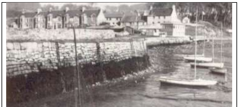
Figure D.2 Bucehaven Pier From Graham (1968)
