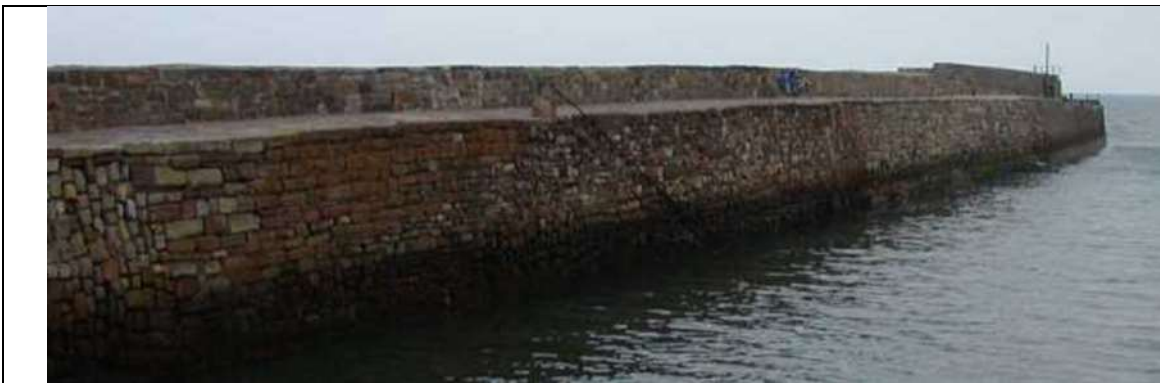
Figure D.10 St Andrews main breakwater showing variable wall construction, July 2003
