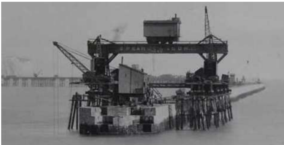
Figure 12.12 Dover - placing concrete blockwork from travelling cranes
