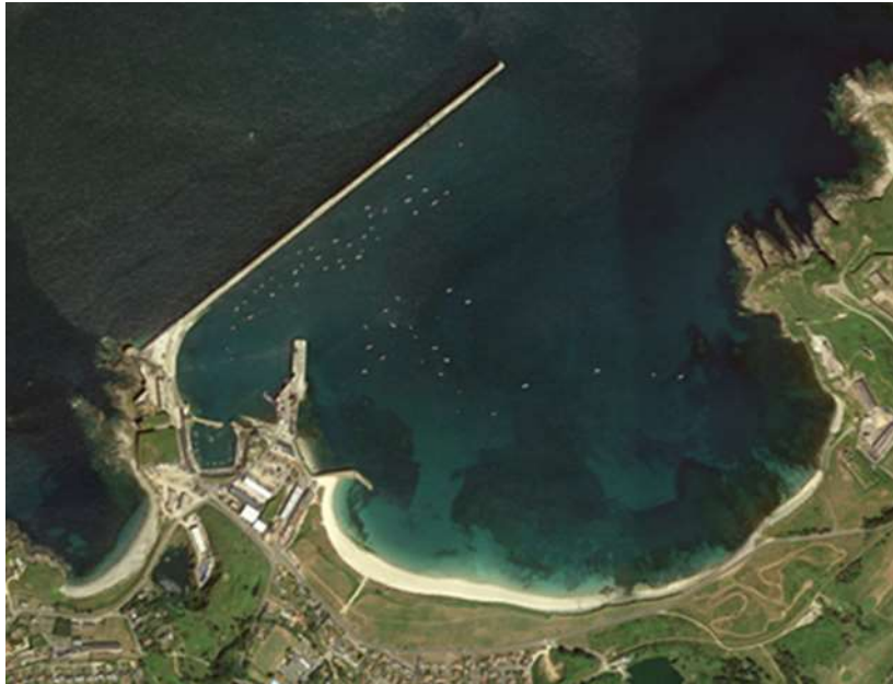
Figure 6.12 The Admiralty breakwater in 2014
