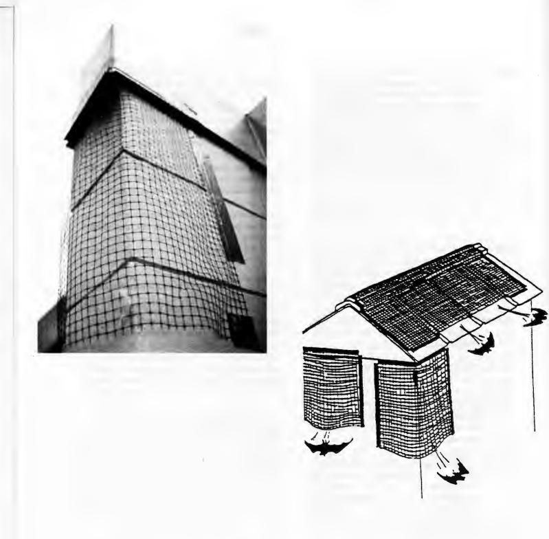
Figure 1. Plastic industrial birdnetting ( $\frac{1}{2} \times \frac{1}{2}$  inch mesh size) used to exclude bats from buildings (a) can be used in many situations (b).
