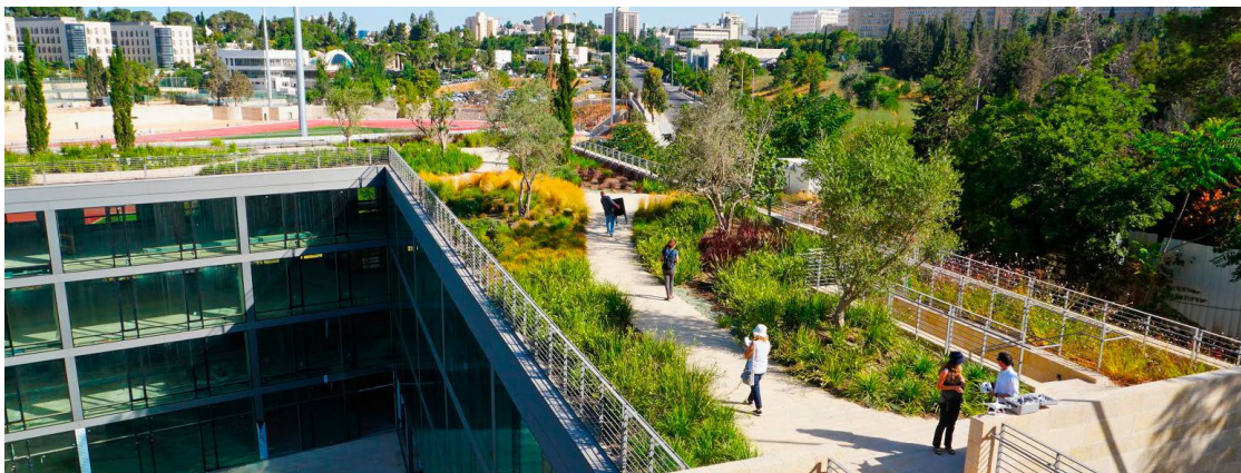
Fig. 1 - Tetto verde intensivo realizzato al “National Campus for the Archeology of Israel” (Source: Zinco Green Roof Systems)
