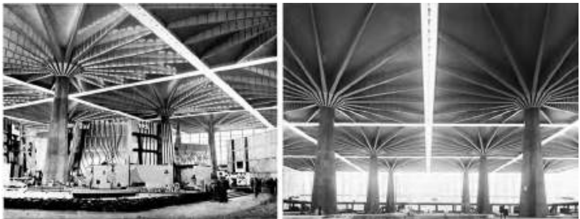
Fig. 3. The Palace of Labor, exhibition of 1961 (NS) and Fig. 4. The Palace of Labor under construction (TSLF).
