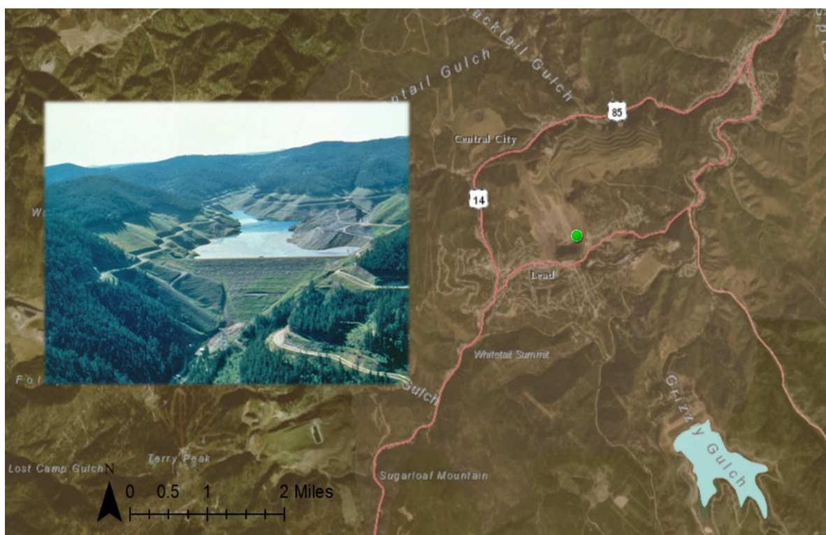
Figure 3.3. Grizzly Gulch Tailings Containment Facility, Lead, SD.
