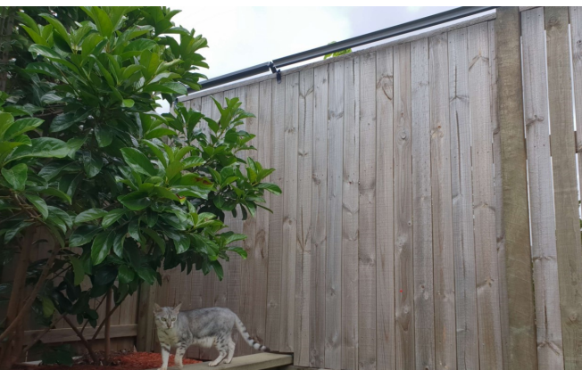
Figure 5. Oscillot® system for preventing cats from climbing over fences.
