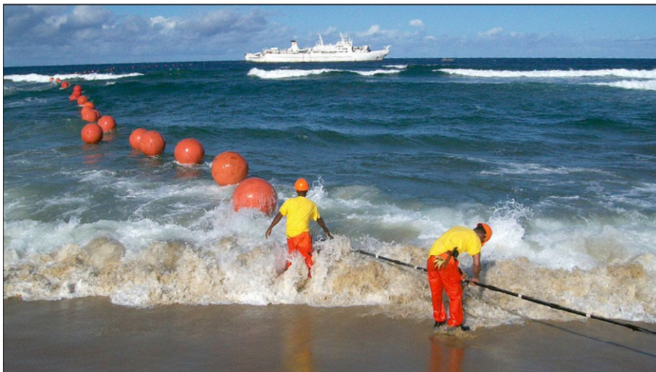
FIGURE 4: CABLE LAYING
