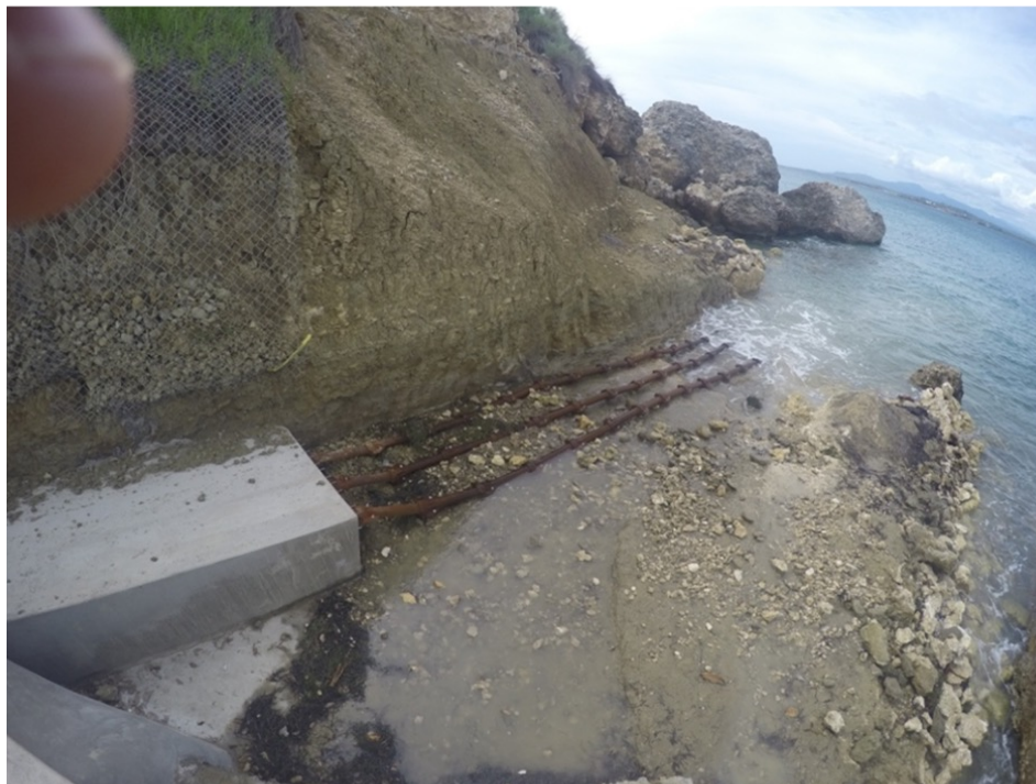
FIGURE 8: GUANTANAMO BAY CABLE LANDING SITE
