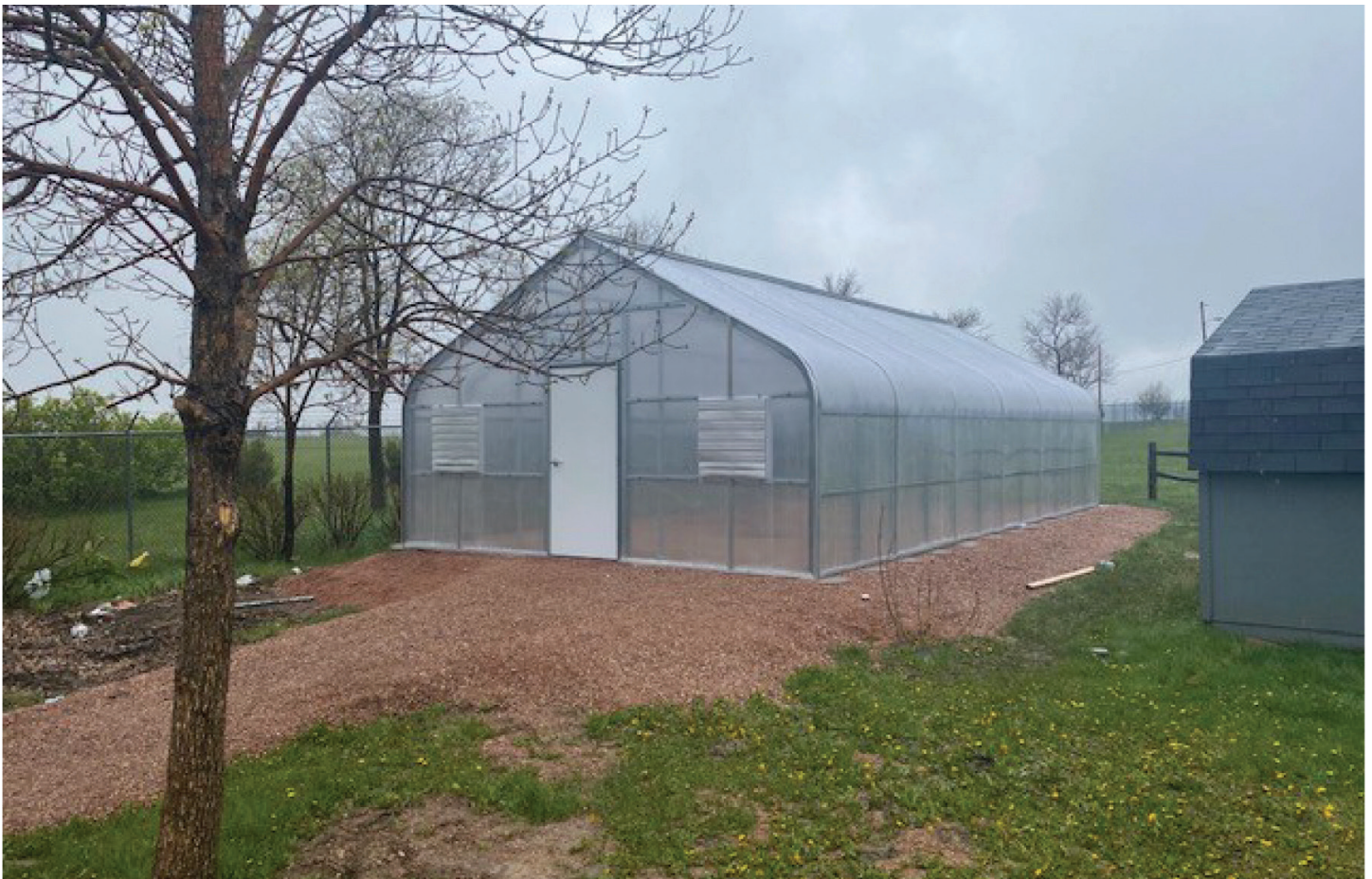
Figure 3. The fully constructed greenhouse in May 2020.
