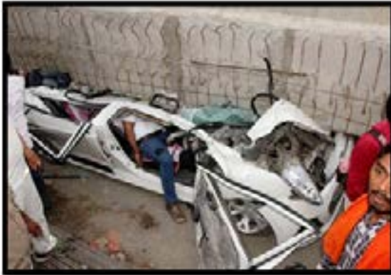
Figure 2. Falling down of Bridge pillar at Cantt, Varanasi
