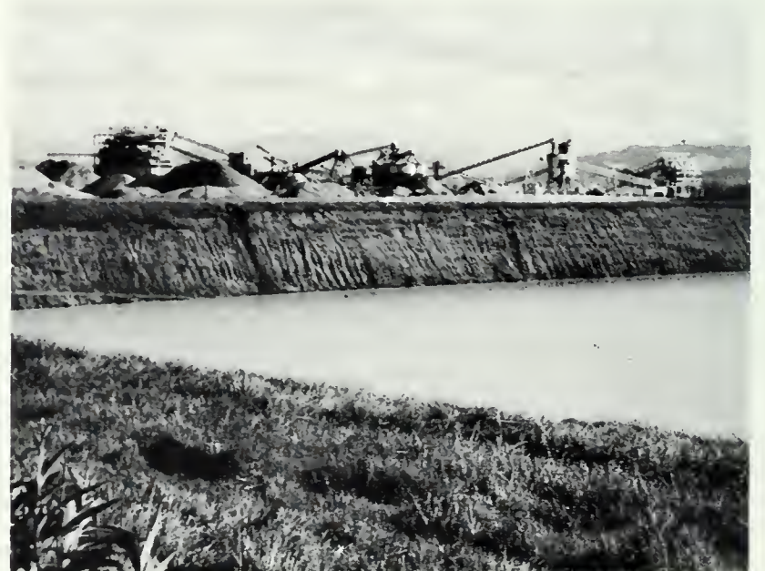
Figure 60 — Making a visual survey of the operating site concerns viewpoints of the public spectator
