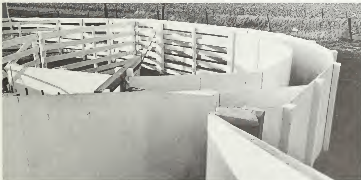
Cattle move through a curved alley better than through a straight alley because they cannot see what is ahead of them. A swinging gate is used to guide cattle into the head catch or up the loading chute. (Fig. 9)
