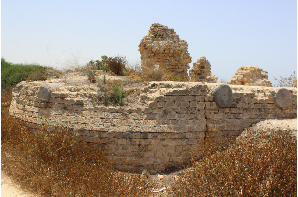
fig. 11. Granite column shaft employed in the tower closed to the Jerusalem Gate (photo author, June 2019).
