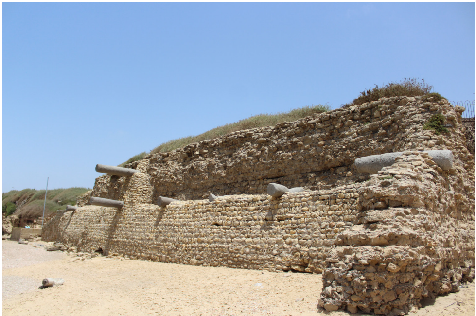
fig. 10. Column shaft used to reinforce the city walls toward the sea (photo author, June 2019).
