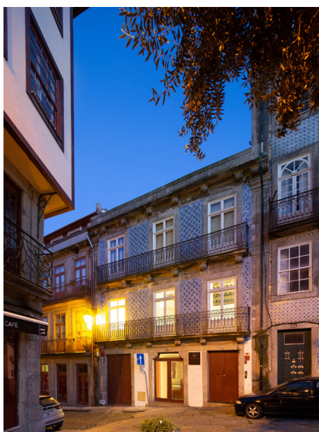
Figura 35. Fachada Typographia Cowork
