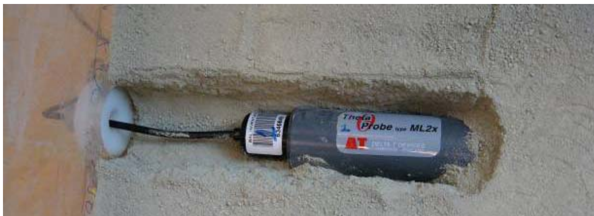
Fig. 4. Installation of the ThetaProbe (TP) sensors
