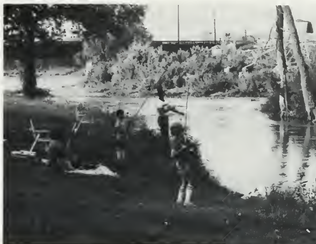
Fig. 8. — Family fishing is important where access is easy, as along the side channel in Wilmington Park.
