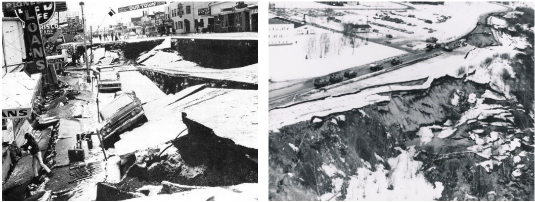
Figure 2.1. Lateral spreading phenomena during Alaska earthquake (1964).
