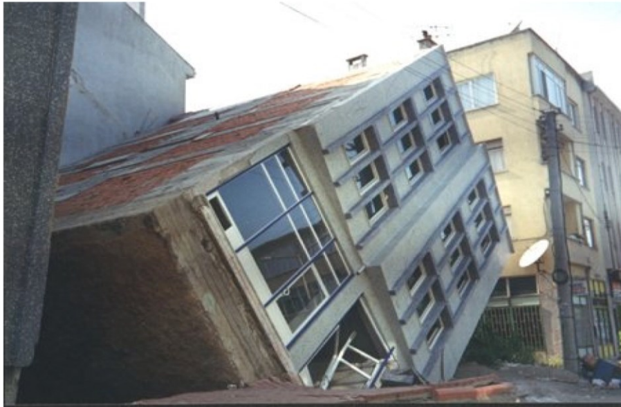
Figure 2.4. Tilting due to liquefaction in Adapazari during Kocaeli earthquake (1999) (Turkey).
