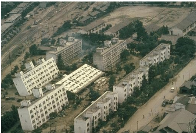
Figure 2.2. Bearing capacity failures during Niigata earthquake (1964).
