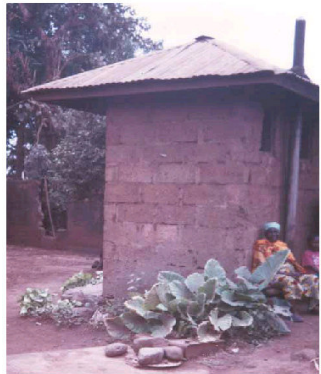
High standing latrines (VIP)
