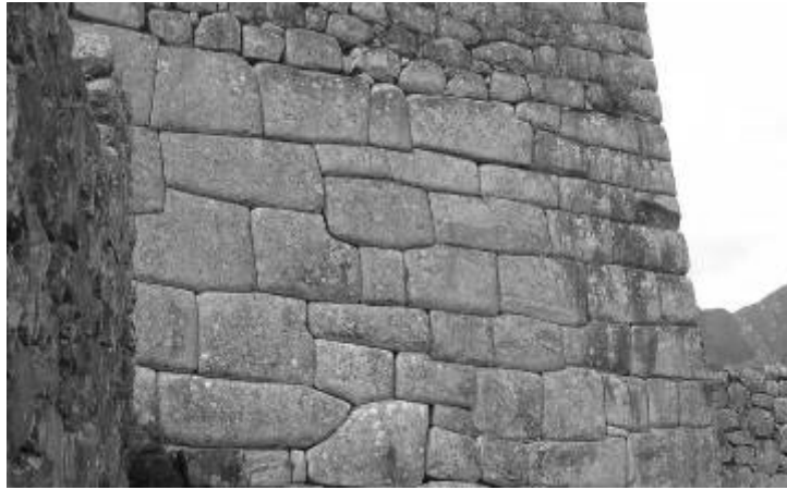
Figure 2. Interlocking blocks at masonry wall in Peru. (Photo: I.Vardoulakis 2006)
