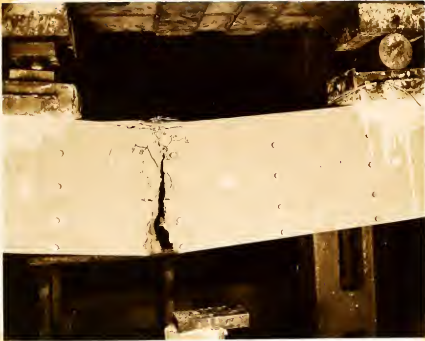
FIG. B20. VIEW OF BEAM B3 AFTER FAILURE
