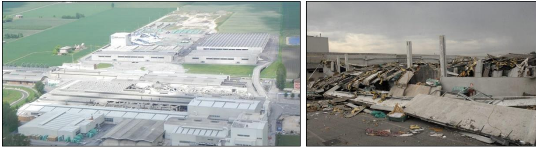
Figure 6-6 Example of industrial buildings in the district of S. Agostino and observed collapse.
