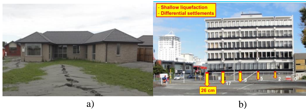
Figure 5-33 Type of damage on wooden; and (b) reinforced concrete buildings (from Cubrinovski et al., 2011c) (the yellow arrows in figure b represent the settlement distribution along the building).
