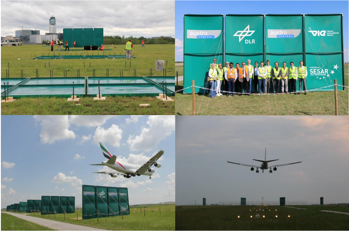
Fig. 4 Impressions of the installation of plate line 2, the visitors' day, and overflights of plate line 1 (in clockwise order).
