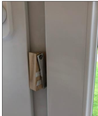
Figure 12: Insertion of cable ties in the window frame
