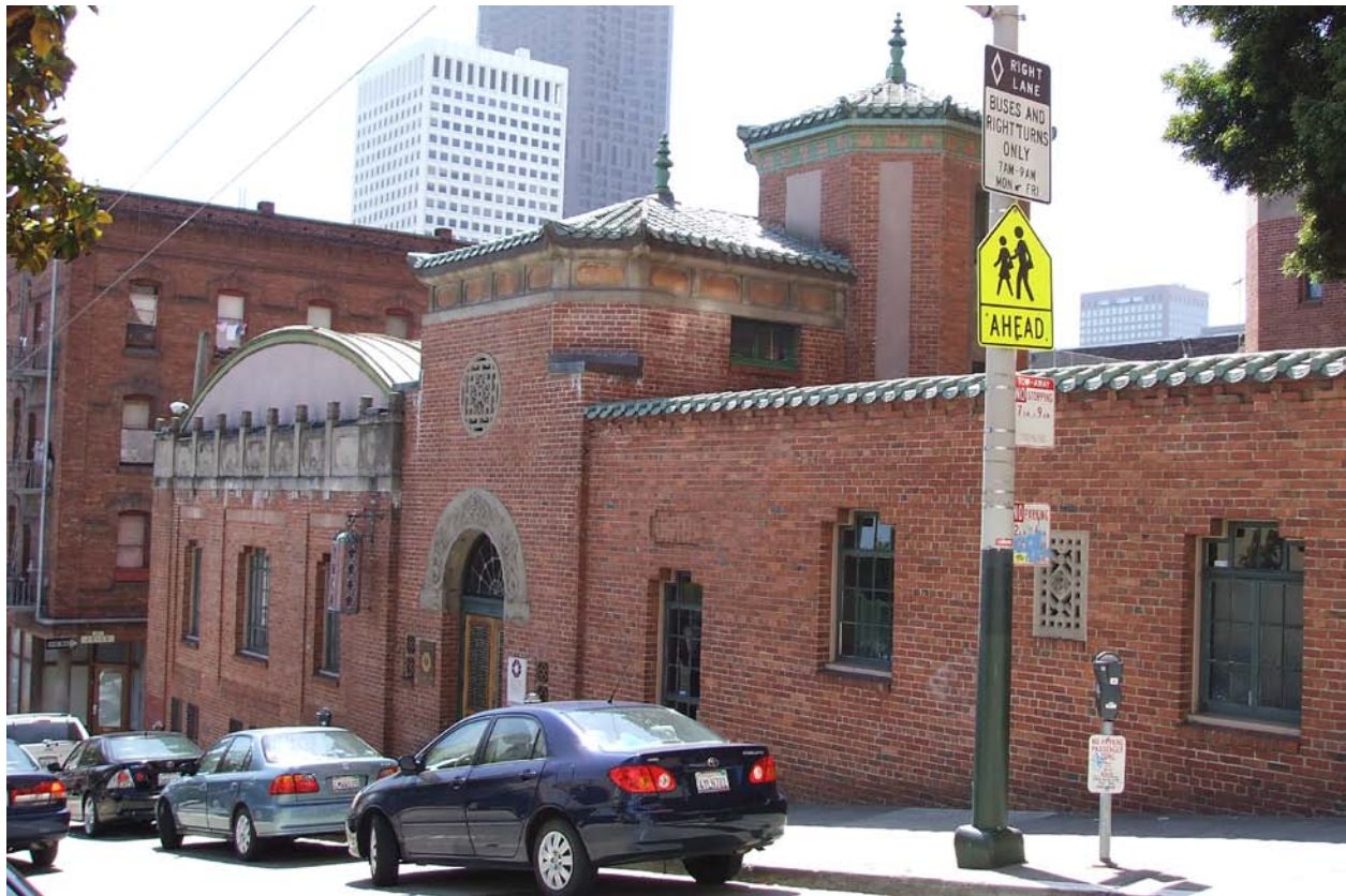
Figure 37: The Chinese YWCA building, now is used as the Chinese Historical Society of America Museum and Learning Center, ca.2007 (Photo by author).
