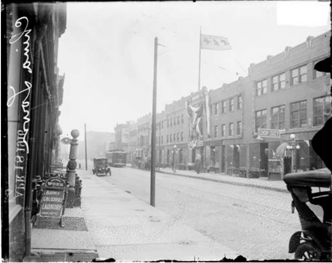
Figure 18: View of 22 nd Street (Cermak Road), ca. 1916 (Source: Chicago Historical Society)
