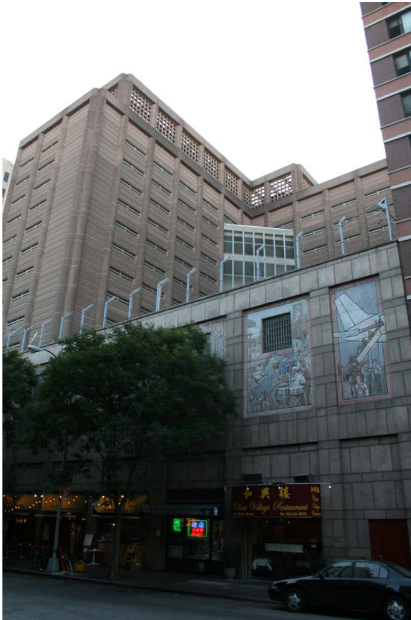
Figure 31: The White Street Jail with its lower levels facing Baxter Street used for commercial and community space, ca. 2008 (Photo by author)
