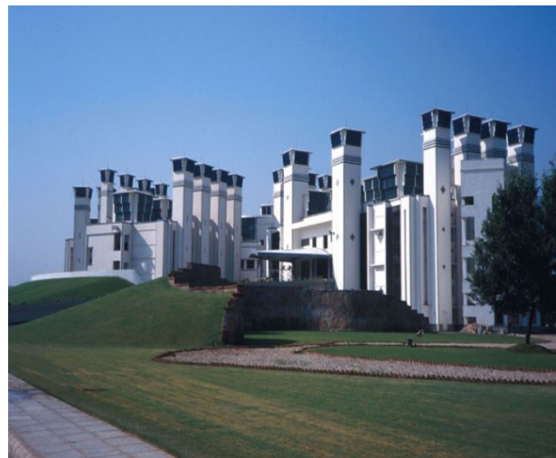
Figure 2.5 Torrenet Research Center (Source: Website, http://archnet.org )
