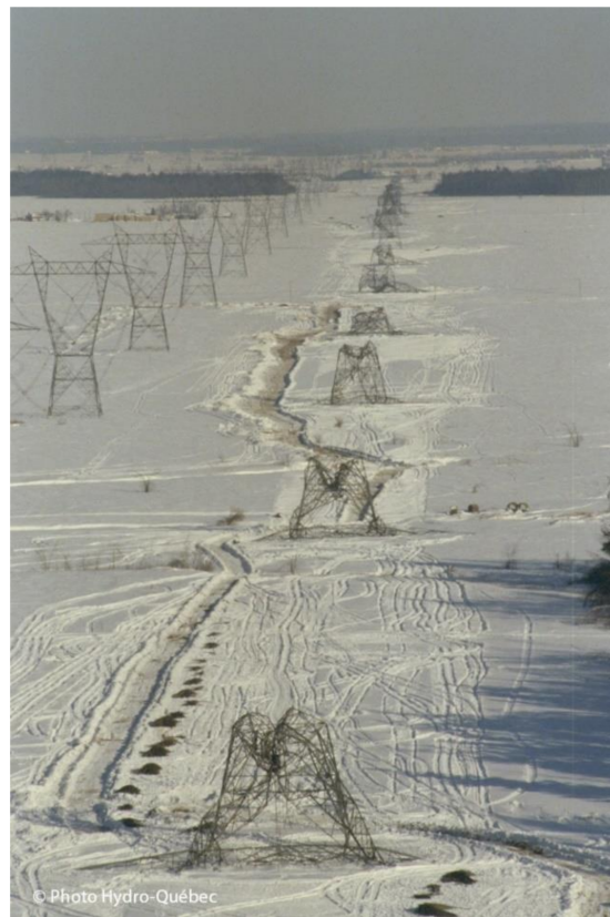
Figure 1. Example of icing impact on a high voltage transmission line (1998 Eastern Canada ice storm, credit: Photo Hydro-Québec).
