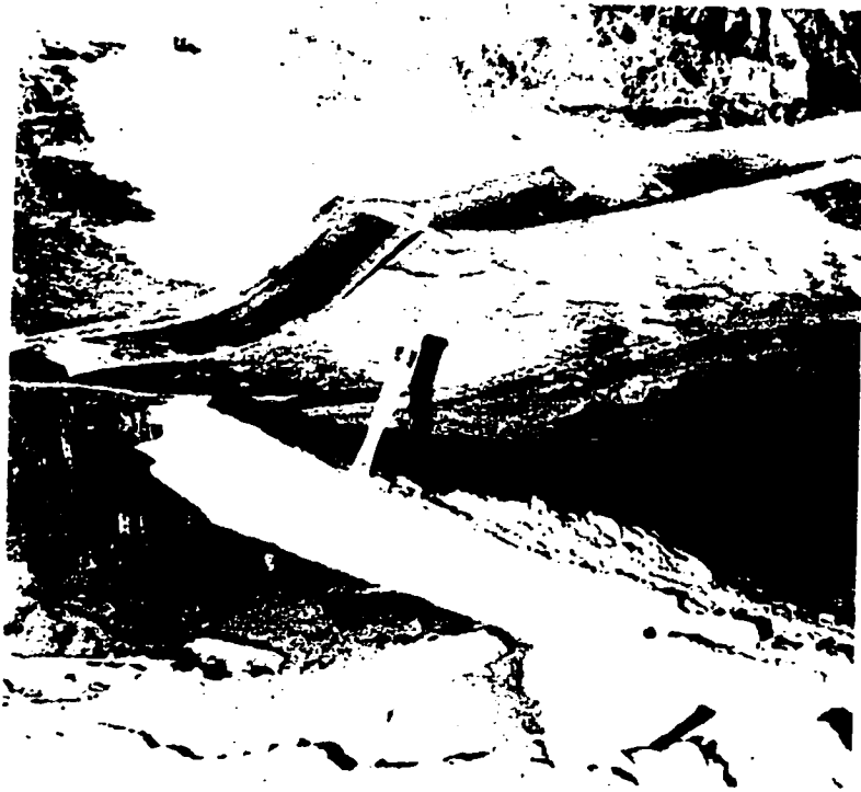
Fig. 1.4 Floor heave at the center of an entry at the Glen Rogers Mine (after Aggson, 1978)
