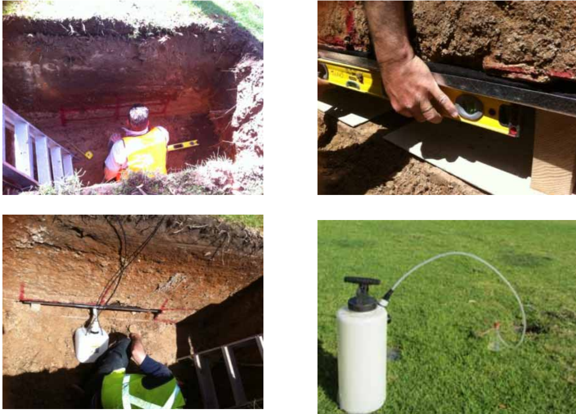
Figure 2. Lysimeter installation
