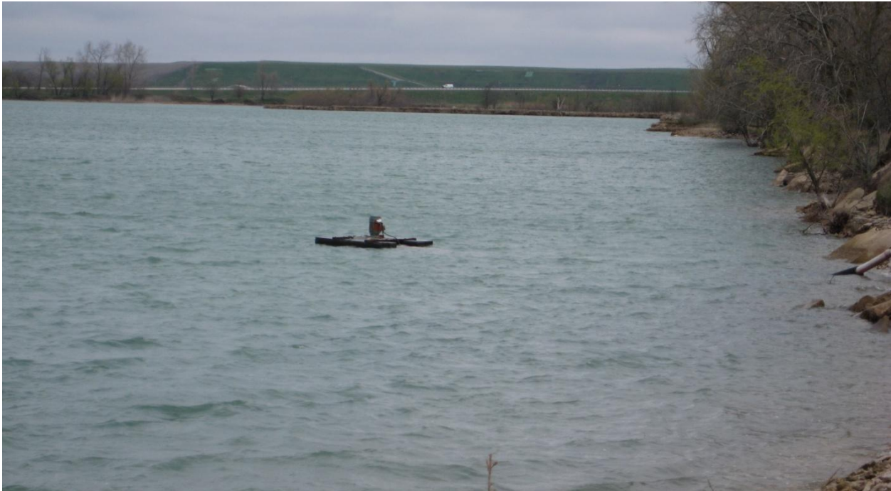
Figure 2.8: A floating pump directs water from the northwest sub-impoundment in the northern basin to the southern basin
