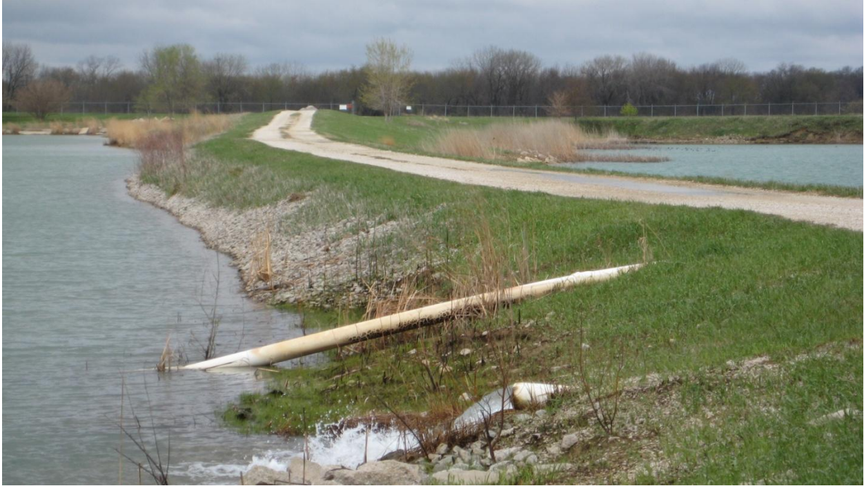
Figure 2.7: Water from the northern is being pumped into the southern basin
