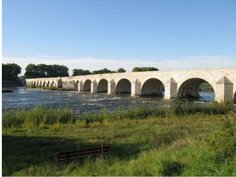
FIGURE 1.22 – Pont de Beaugency sur la Loire [2]
