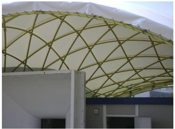
Fig.1. First prototypes of composite materials gridshells at Ecole des Ponts ParisTech
