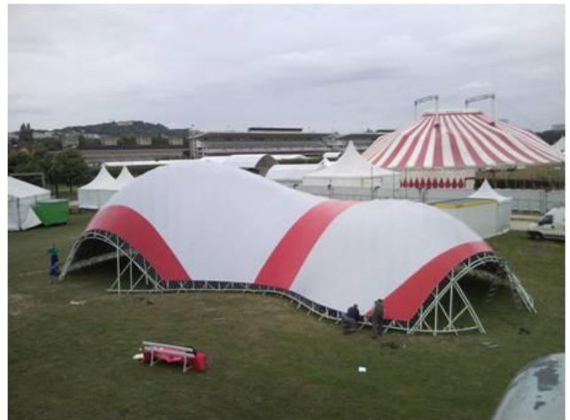
Fig. 2. Gridshell in composite materials for Solidays festival in Paris
