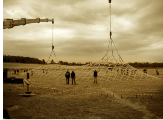
Figure 2: Grid erection.
