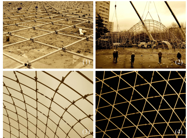
Fig. 6. Assembly (1) | Erection (2) | Erected grid (3) | Braced grid (4)
