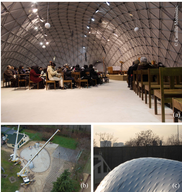
Fig. 1. Interior view (a) | Grid erection (b) | Exterior view (c).
