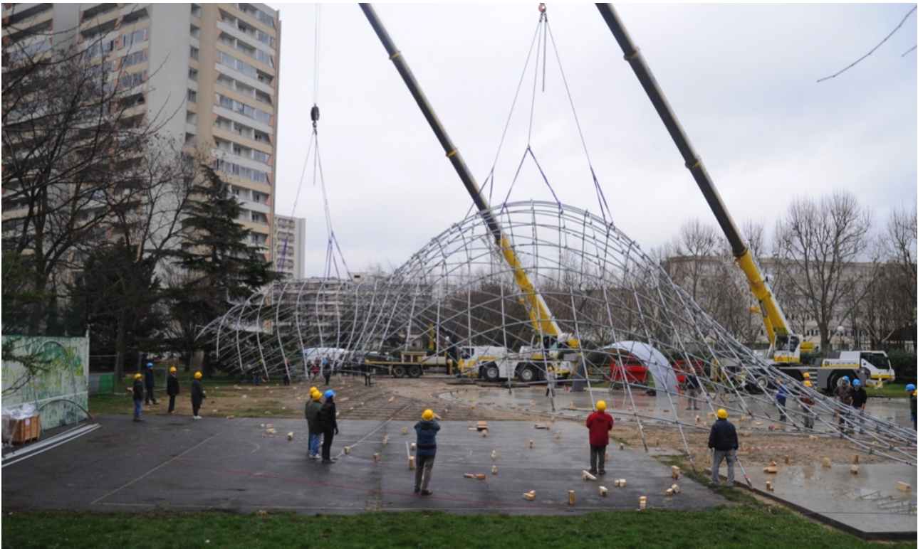
Fig. 5 Erection of the primary grid by two cranes
