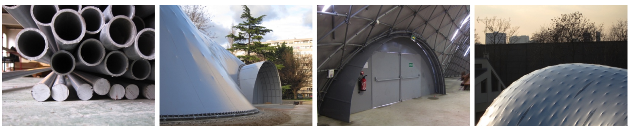
Fig. 2 GFRP tubes, steel door, grid, PVC coated fabric
