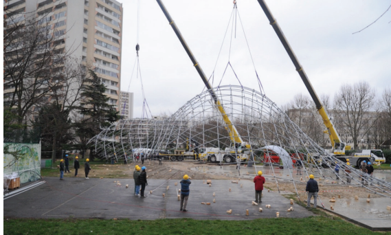
Figure 2: Grid erection with large deflections
