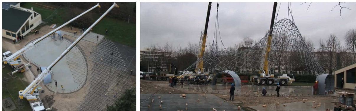
Figure 1. Cathedrale Ephemere de Creteil. a. Primary grid made flat. b. Primary grid deformed elastically and attached to boundary conditions.
