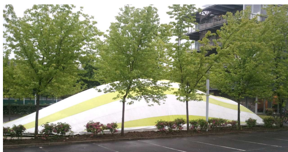
Figure 4: Long term erected composite gridshell. Some planar parts (yellow) of the membrane can be seen.
