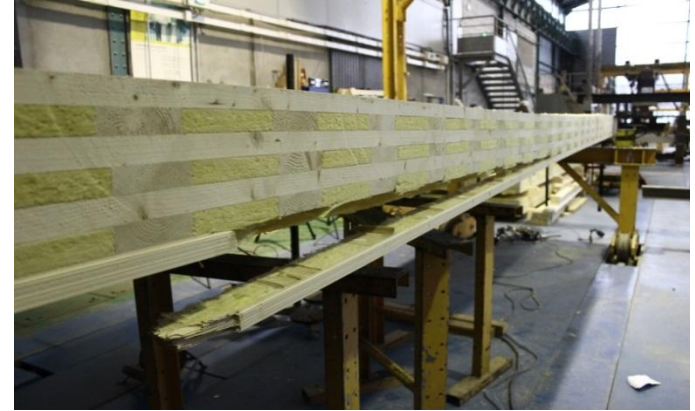
Panobloc ® 2/3, less spaced: tensile failure of bottom boards
