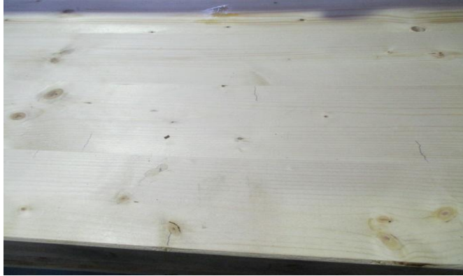
Massive CLT panel: ductile longitudinal compressive cracks before tensile failure
