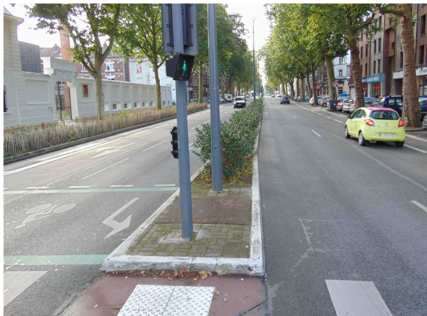
Figure 4: Thorn bushes in the middle and lateral fences on Montebello boulevard in Lille to prevent straight line pedestrian movements towards the entrance of Wazemmes secondary school (left) and channel them on safe pedestrian crossings, renunciation to the principles of legibility and openness of space design (Photo L'Hostis 2014)
