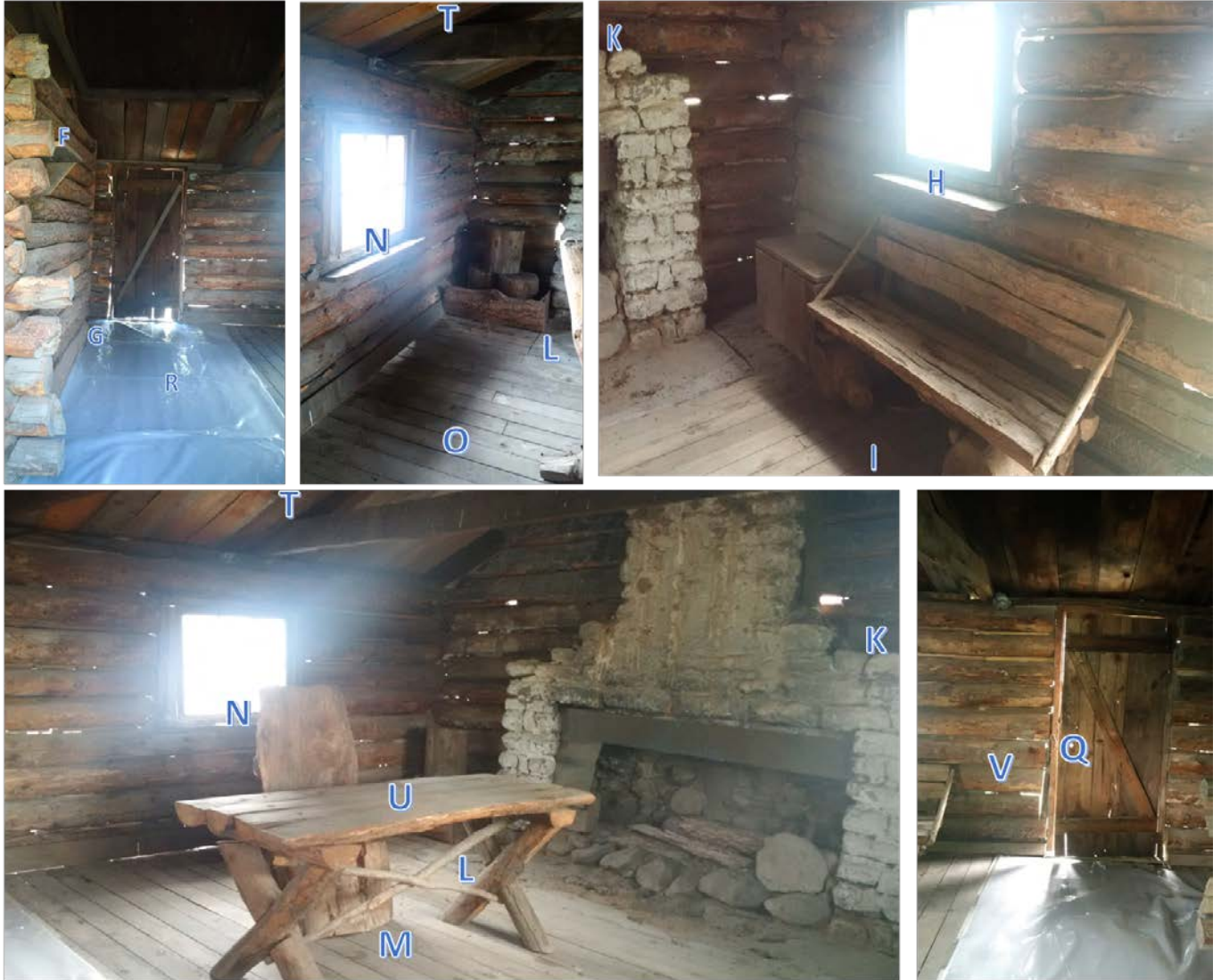
Top left: view of the west entrance. Top middle: view of the west side of the cabin. Top right: view of the east side of the cabin. Bottom left: view of the main room and west and north side of the cabin. Bottom right: view of the east entrance.
